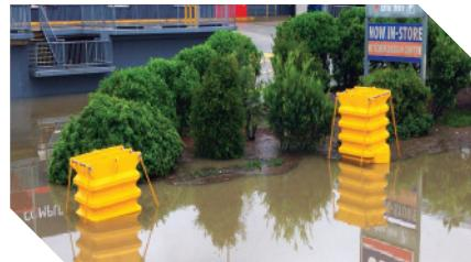
Compact and easy to install, Flood Tuff units can be stored locally and deployed quickly, even in challenging conditions. In 2025, 25 Flood Tuffs were deployed in Brisbane during Cyclone Alfred. Despite five of the sites reaching up to 1.6m floodwater depth, Flood Tuff successfully prevented any water damage to the equipment contained within.
