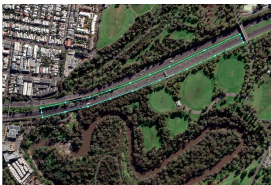
(a) Case A: M3 Freeway towards city
